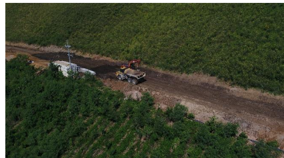
Image 5. The use of FABA as Roadbase material [7]
