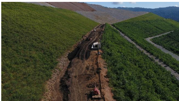
Image 5. The use of FABA as Roadbase material [7]
